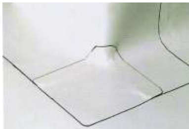
Outside corner treatment
